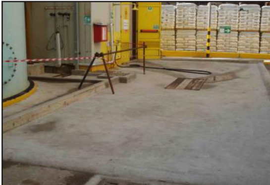
Concrete slab following surface preparation
