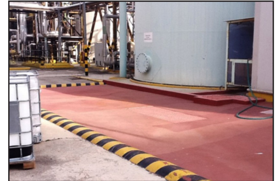
The area 6 years after installation
