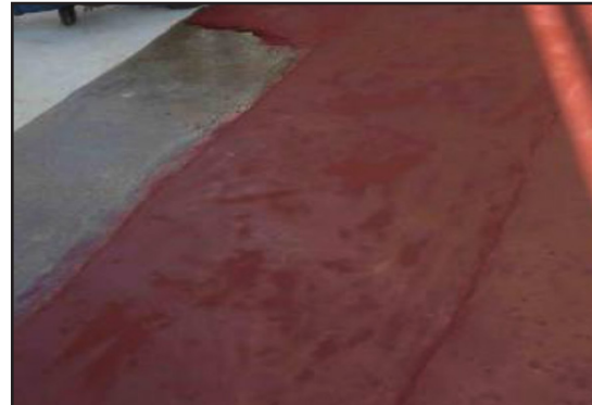
ARC 988 being trowel applied
